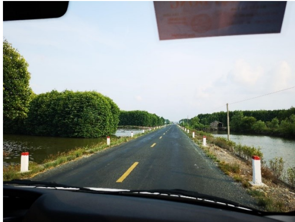
Fig. A.1 Elevated roads in Ca Mau province
