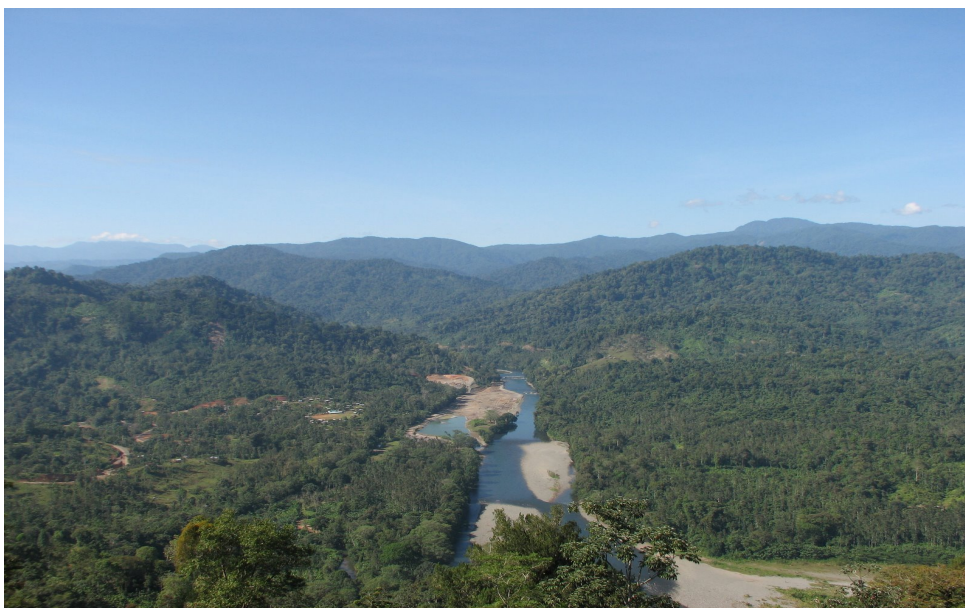
Fig. 47: LAPBR: Changuinola river in Palo Seco Protector Forest (Buffer zone), 6 km downstream of the beginning of construction of Dam Chan 75 in Dec. 2007. Photo: A. Rodriguez
