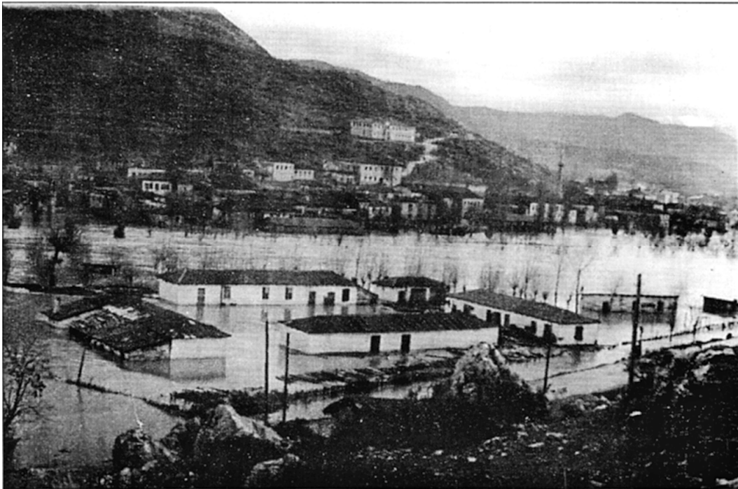
Photo 6: Flood event from January 1963, inundating the town of Lezha (Photo: Pulaha & Parruca, 2006: 131).
